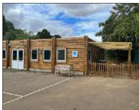
PURPOSE-BUILT: The Cabin at Gamlingay has been completed.
